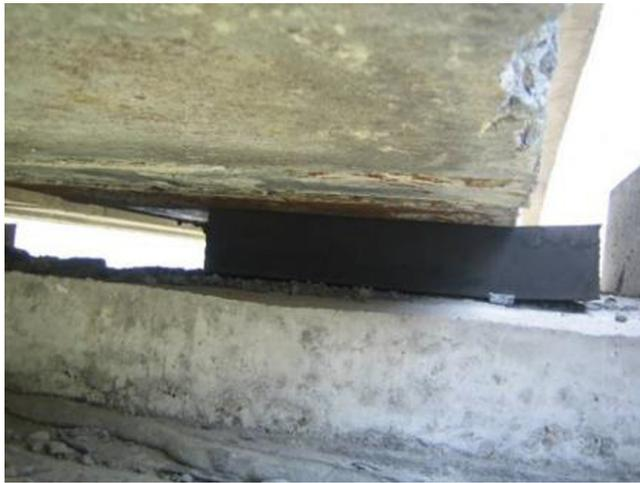
Fig. 2. Sliding of laminated-rubber bearings.
