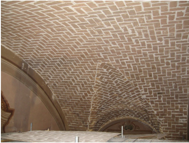
Fig. 1. Typical single leaf vault with herringbone brick pattern.
