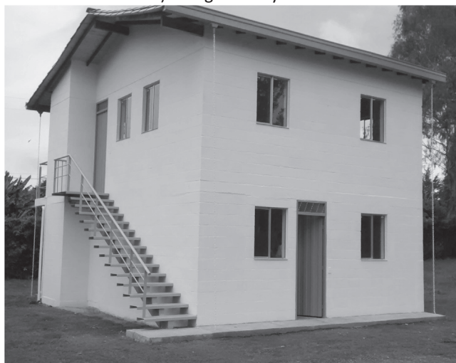
b) Two-story building
