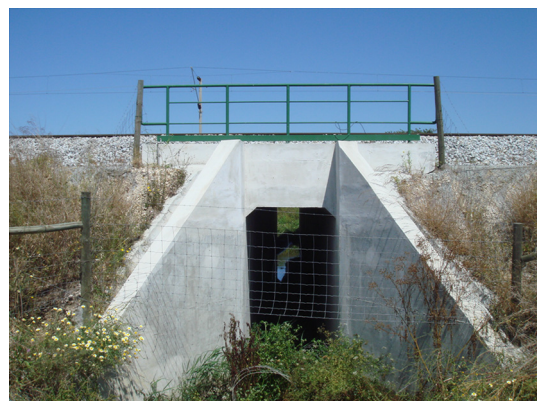
Fig. 1. Culvert transition PH126A.
