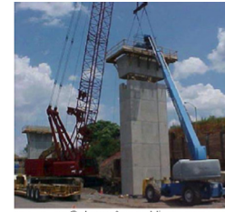
Column Assembling
