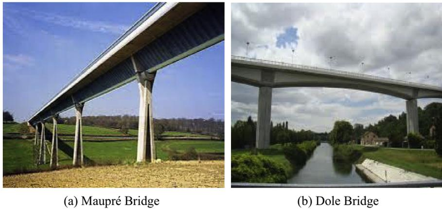
Fig. 1. Plate girders with corrugated webs: (a) prismatic and (b) tapered plate girders [10].
