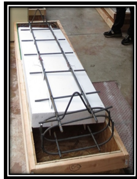
Fig. 4. Assembly with segmental FRP connector.
