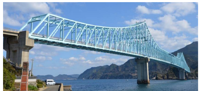
Fig. 2. Photo of the bridge.
