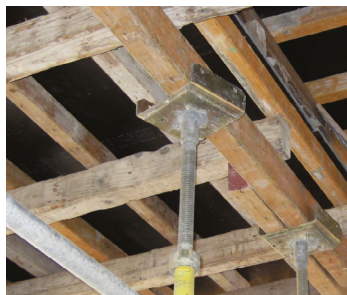
Fig. 2. Timber bearer supported by U-head jack.
