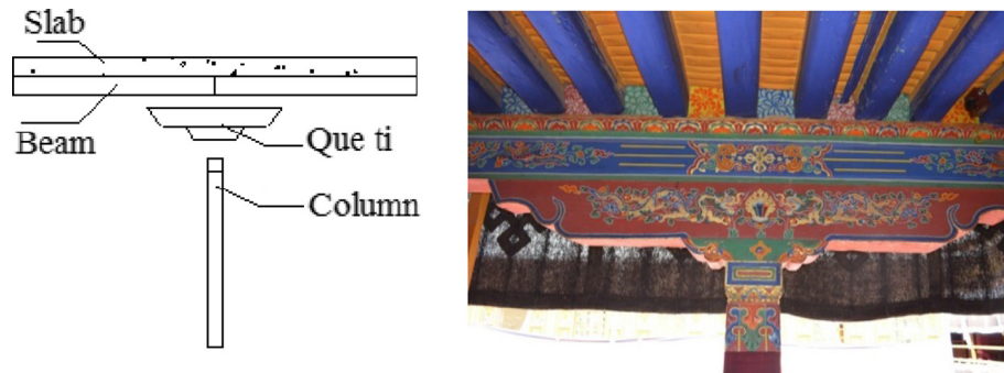
Fig. 1. Composition of beam-column joints.
