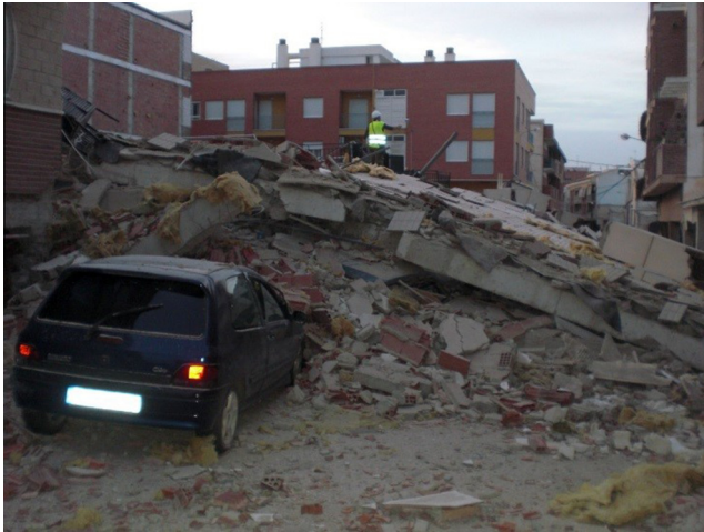
Fig. 1. Building failure in Lorca earthquake (Spain, 2011).
