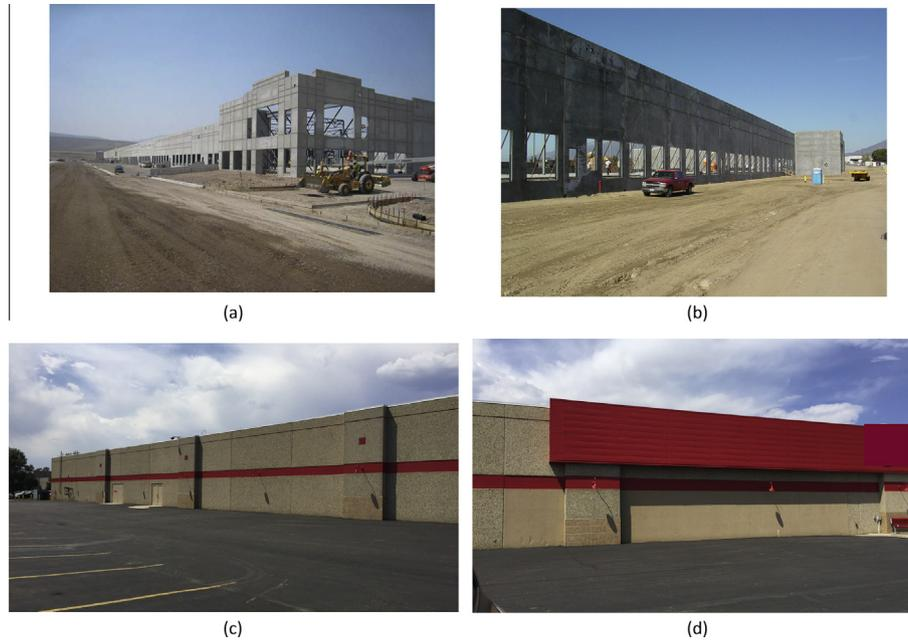
**Fig. 1.** (a) and (b) Photographs of typical RWFD building construction process in the US (photo credit: J. Lawson), (c) and (d) photographs of typical RWFD commercial buildings (photo credit: J.W. van de Lindt).
