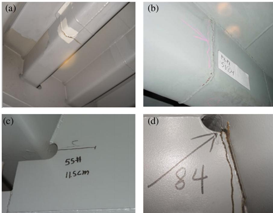
Fig. 2. Observed cracks in orthotropic steel decks located at: butt joints in longitudinal ribs (a) (from Ge and Xiang [7]) and (b) (from Xiao et al. [15]); scallop cutout (c) and rib to web joints (d).
