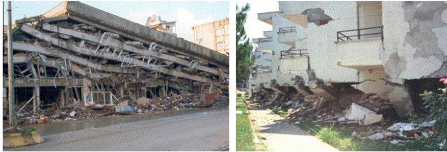
Fig. 1. Strong beam and weak column failures, from [3].
