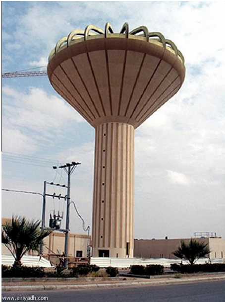
Fig. 1. Reinforced concrete elevated conical tank in Saudi Arabia in Alriyadh News Paper [3].
