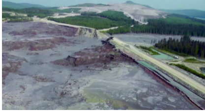
Fig. 1. Illustration of tailings embankment failure-case of the Mount Polley Mine (Cariboo Regional District, Canada, 2014) [1].
