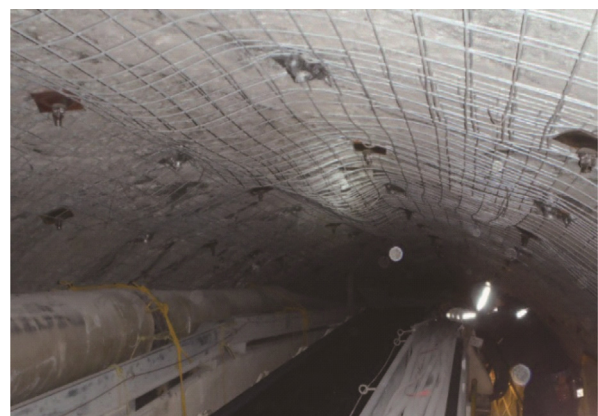
Fig. 4. Drift convergence August 2014 (mesh was installed tight to rock surface).
