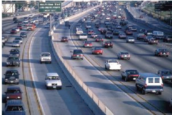
Figure 1. Buffer-Separated HOV lanes with tall median barrier.
