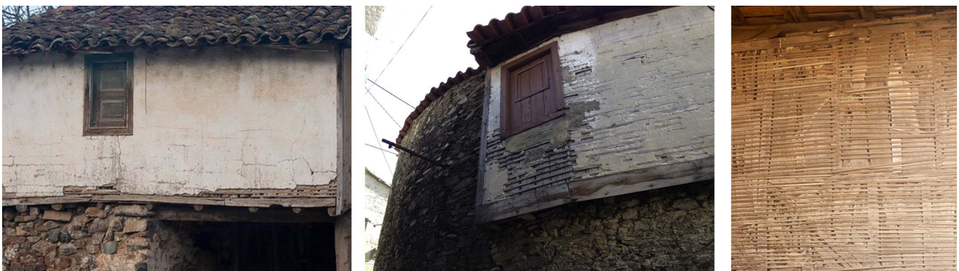
Fig. 1. Tabique wall building details.
