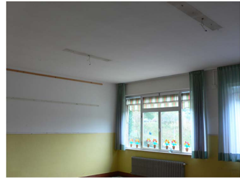
Fig. 3. One of the classrooms on the ground story. The photo also shows the drop ceiling, which allowed the new transverse beams to be covered.
