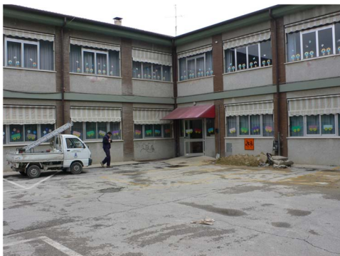
Fig. 2. The school complex is composed of the classroom building, the gym and a porch. Long wing (on the left) and short wing (on the right) of the classroom building: school's backside, which faces onto the courtyard.
