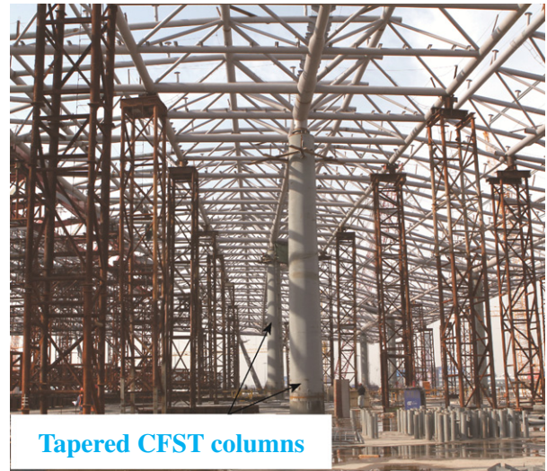
Fig. 1. Tapered CFST columns used in a spacious structure.
