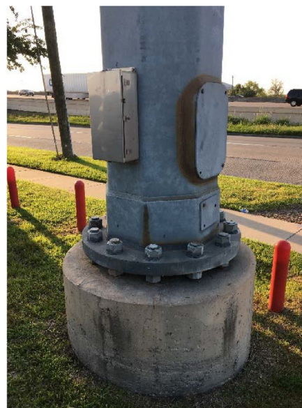
(b) HMIP base connection details
