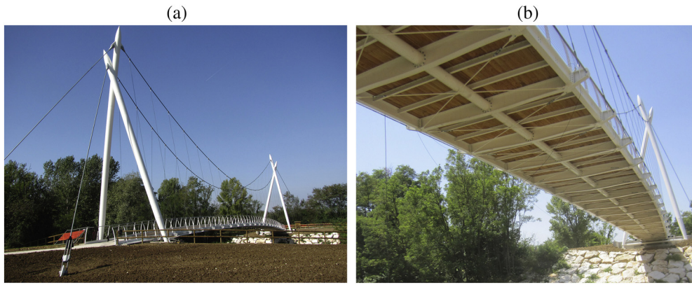
Fig. 1. Footbridge crossing the Serio river (Seriata, Italy): (a) General view; (b) Underside view of the deck.
