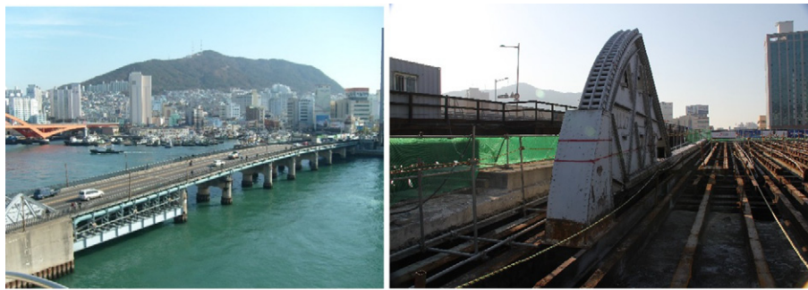
(a) Before and after demolition of the 75-year-old Yeongdo Bridge.
