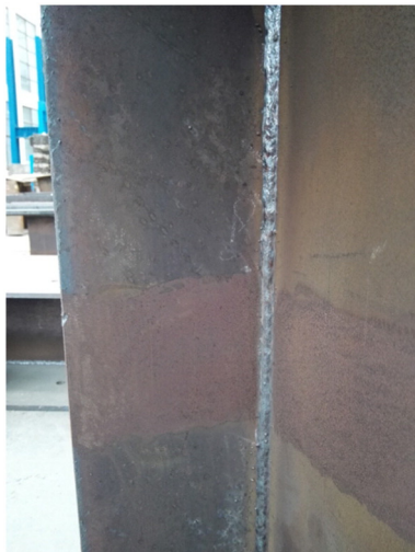
Fig. 2. Specimen ST2 after welding.
