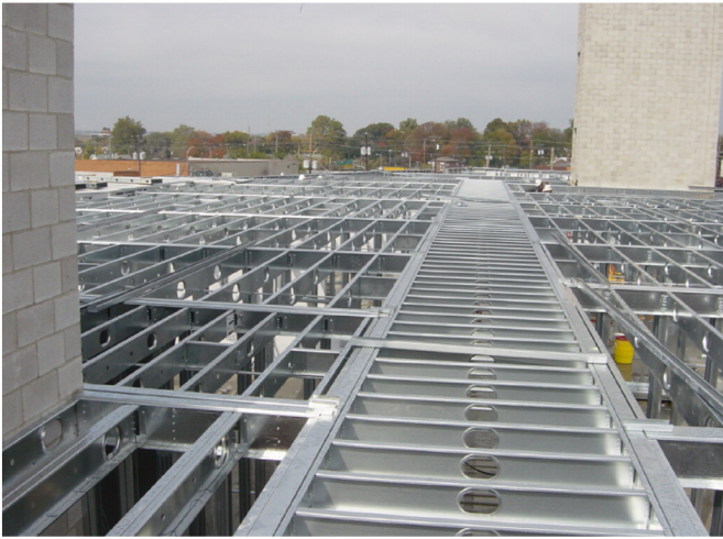
Fig. 1. Cold-formed framing system. (Courtesy: ClarkDietrich Building Systems).
