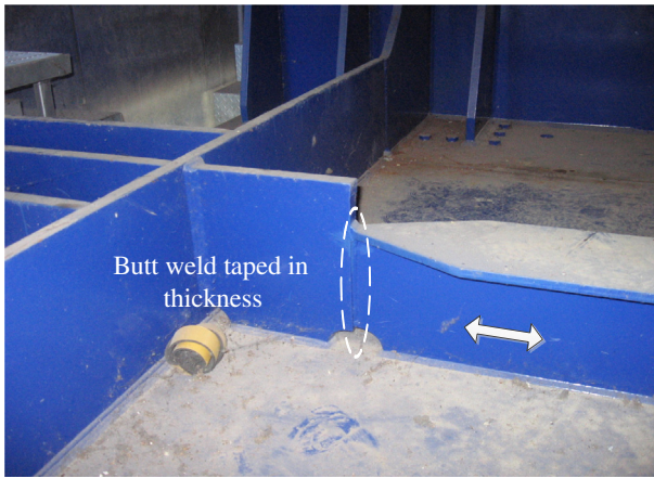
Fig. 1. Typical application of BWSPDT [1].
