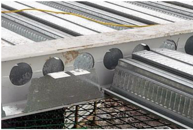
(b) SCCFB with decking configuration
