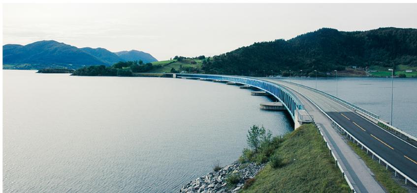
Fig. 1. The Bergsøysund Bridge. Photograph by NTNU/K.A. Kvåle.
