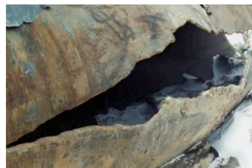
Fig. 1. Burst failure caused by an axial crack in the operation of a pipeline.
