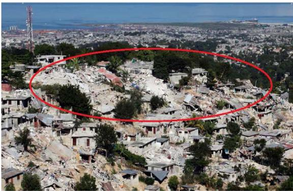
Fig. 1. Destruction pattern on the hill crest following the 2010 Haiti earthquake.
