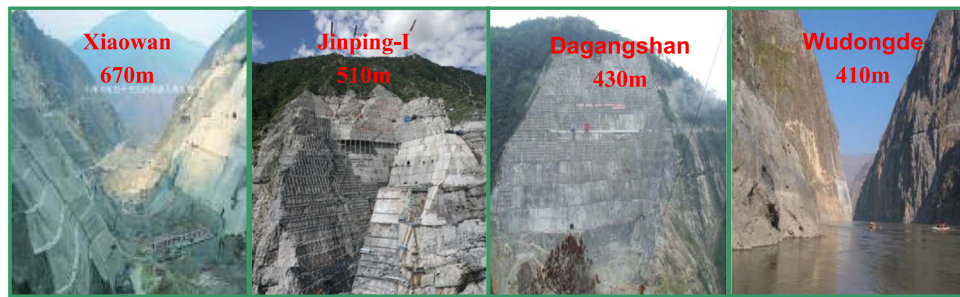
Fig. 1. Typical high dam abutment slopes in Southwest China.
