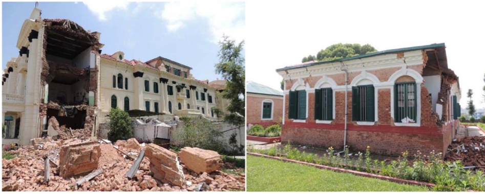
Fig. 1. Recurrent seismic damages in masonry structures (Nepal earthquake, 2015).
