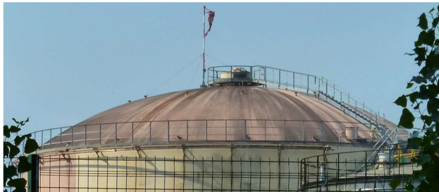
Fig. 2. Typical spherical dome roof on a storage tank.
