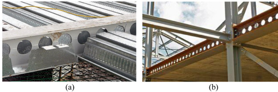
Fig. 2. Shallow cellular floor beam used with (a) profiled steel decking (b) precast floor units (courtesy of ASD Westok Limited).
