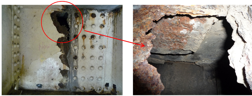
Fig. 1. End cross-girder.
