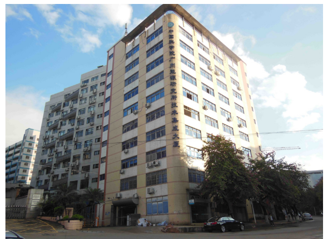
Fig. 1. General view of JCM.
