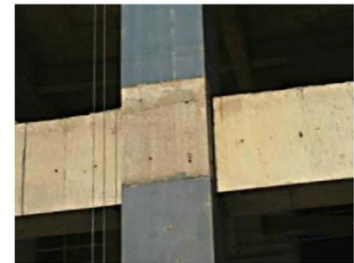
(c) Details of the beam-to-column connection
