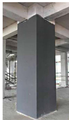
(b) Details of a TRC column
