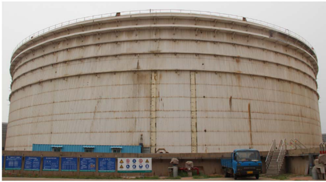
Fig. 1. Selected unanchored open-top oil tank with stepped walls used in the test.
