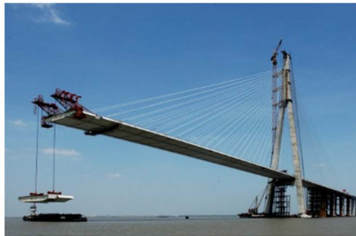
(b) bridge construction
