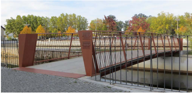
Fig. 1. General view of the St. Mateus hybrid footbridge, Viseu, Portugal.
