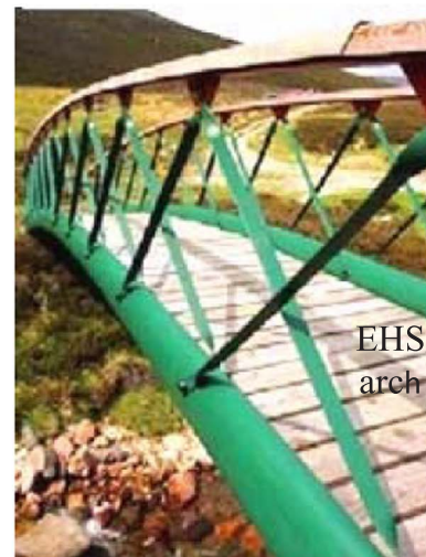
c) Highland Society Bridge in Braemar, UK [12]
