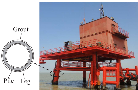
Fig. 1. GFDST used in offshore jacket platform.
