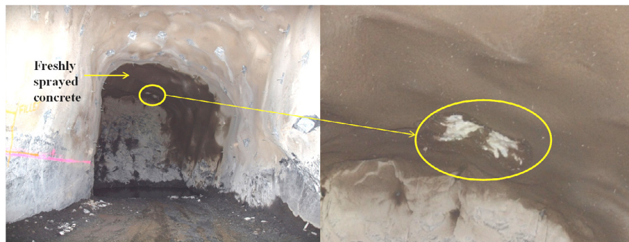
Fig. 2. A freshly sprayed fibre reinforced concrete layer becoming unstable due to its own weight.
