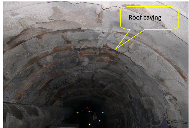
Fig. 2. Roof caving.
