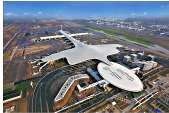
(b) Shenzhen Bao'an International Airport
