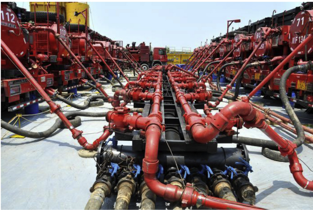
Fig. 1. The high pressure manifolds in fracturing operation.
