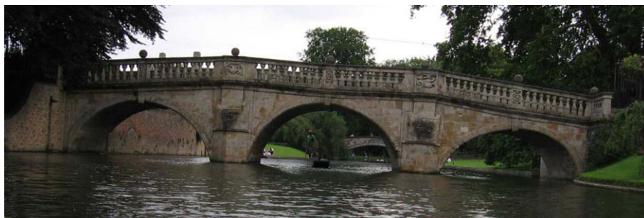
Fig. 1. Clare College Bridge (north façade).
