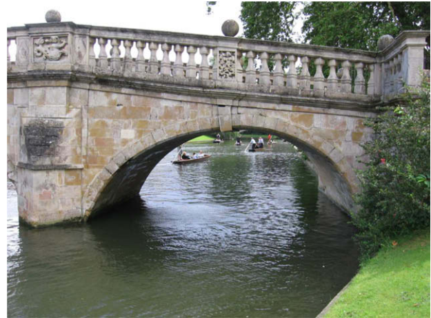
Fig. 2. Clare College Bridge: western span and pier (north façade).
