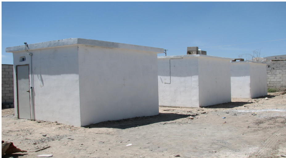
Fig. 1. Test-huts built in Torreón, Coahuila, Mexico.
