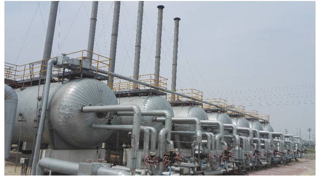
Fig. 1. Horizontal heating furnace in the Daqing petroleum industry of China.
